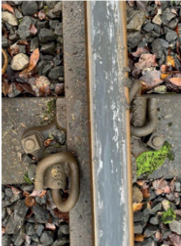
Rails contaminated with leave
