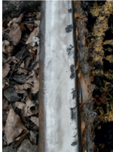
Rails contaminated with grease/lubricant
